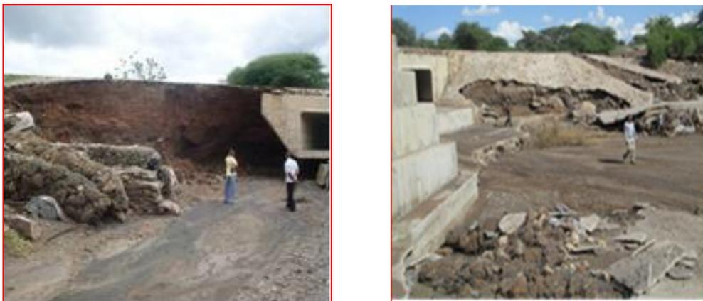
Figure 3 Scouring downstream the culverts due to overtopping
