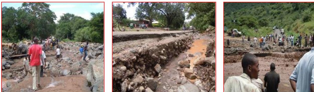
**Figure 2 (a) - (f) Types of flood damages on road elements at Kirurumo Bridge**
